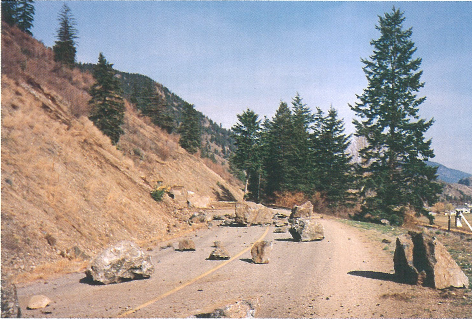
Scattered rocks at base of bedrock bluff
