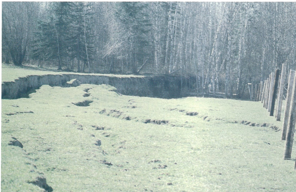
Crescent shaped tension cracks and/or disrupted fence line indicate imminent slope failure
