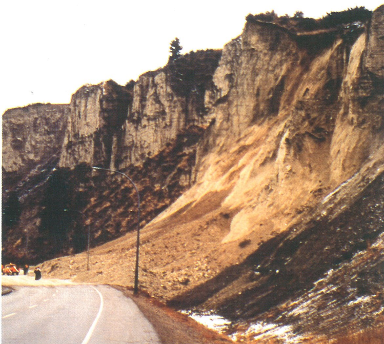
Steep soil face with fresh accumulation of soil at base
