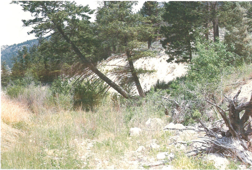
Bulging toe and outward leaning trees indicate a rock or earth slump
