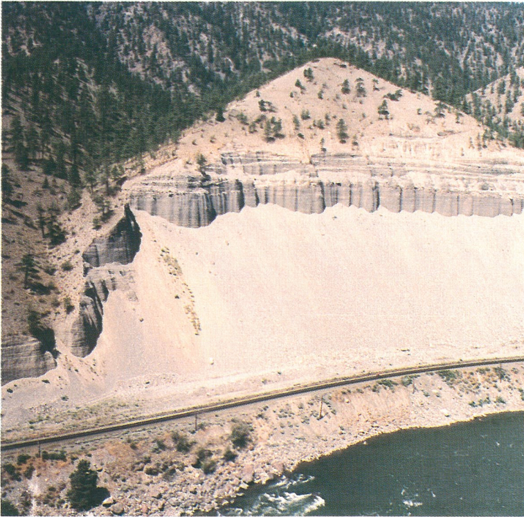
Steep coarse grained soil face with fresh accumulation of debris at base.
