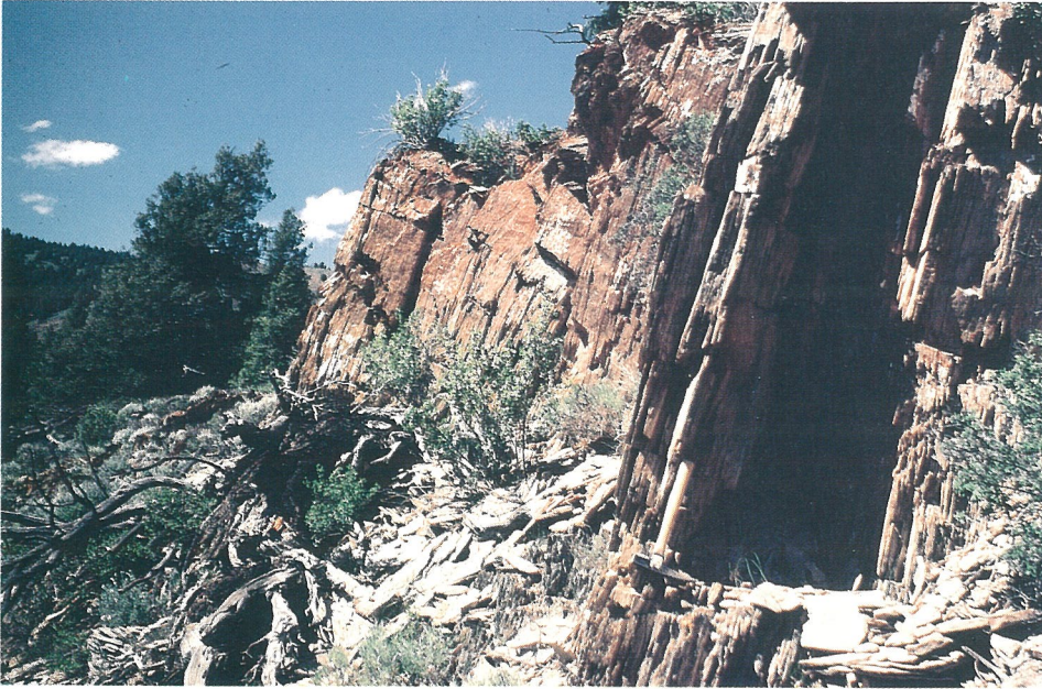
A steep fractured bedrock face can lead to rock falls
