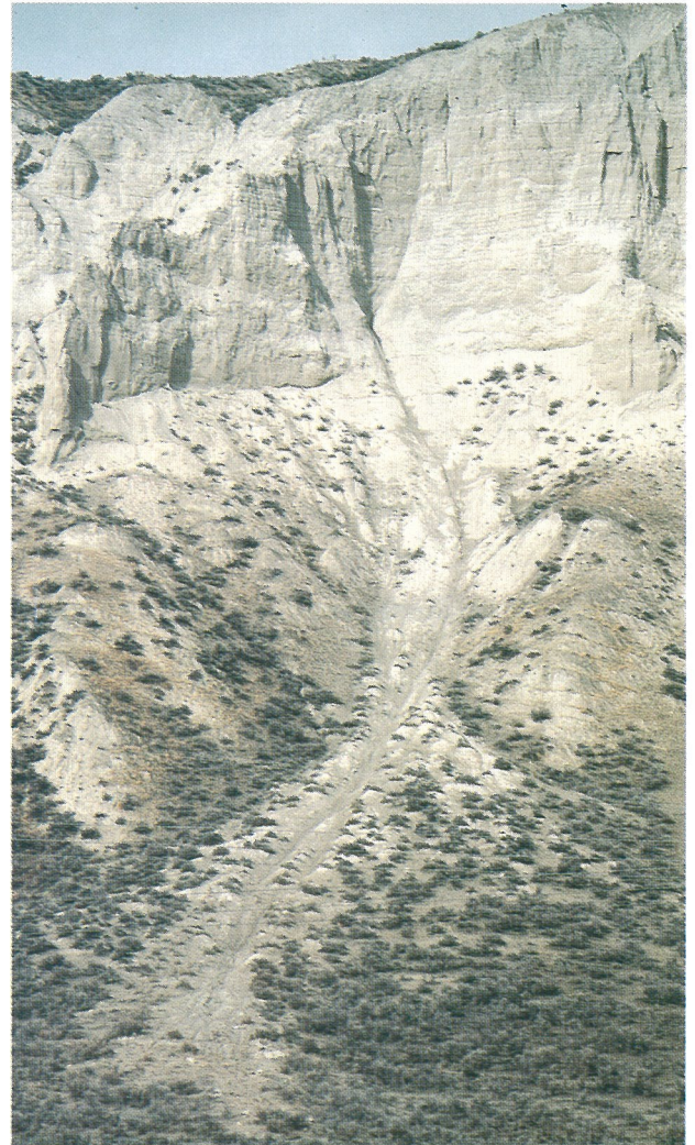
Steep soil face at top of bluff with build-up of soil at base of bluff
