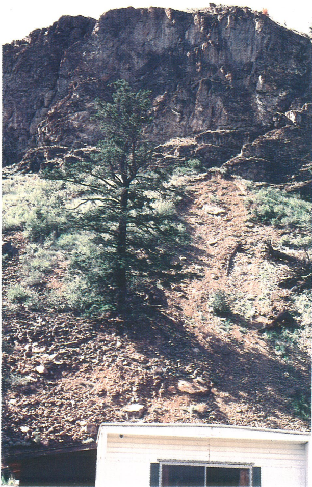
Fractured bedrock face at top of bluff with fresh talus at base of bluff
