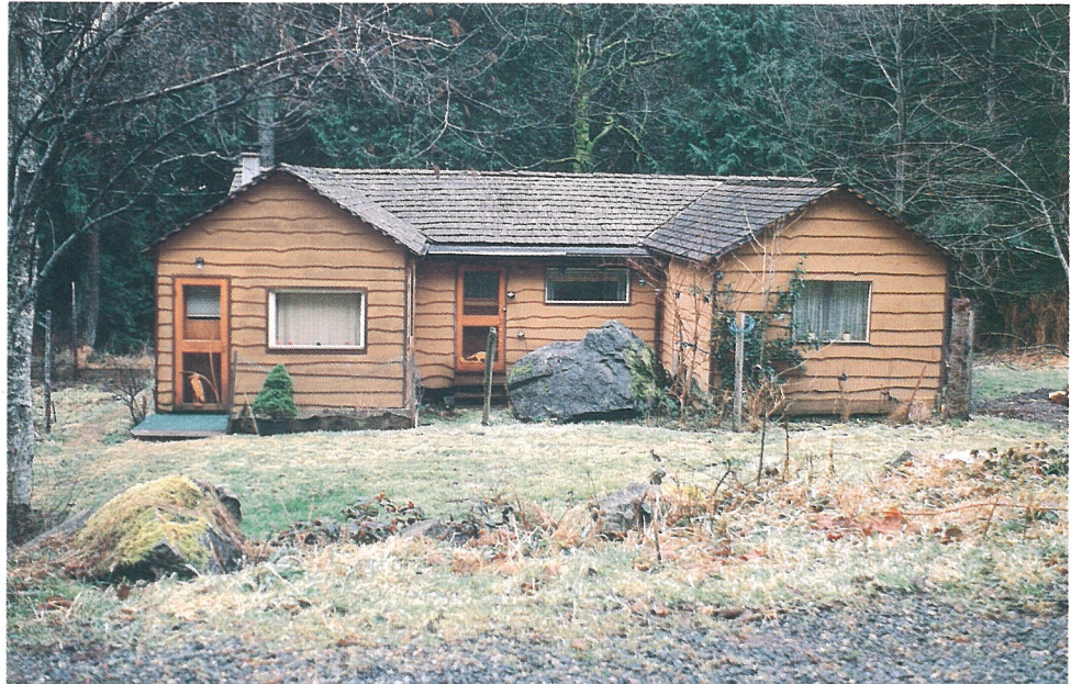
Scattered rock boulders may indicate past rock falls
