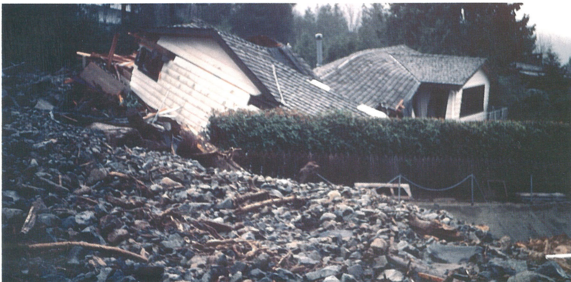
A house destroyed by a debris flow
