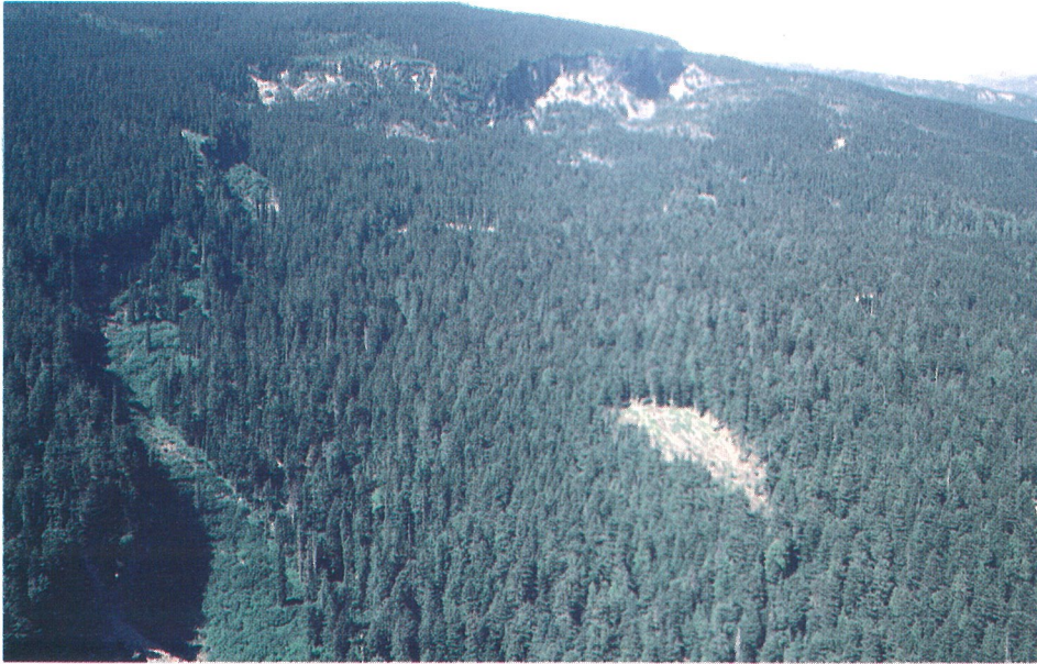
Large crescent shaped headscarp (Downie Slide)
