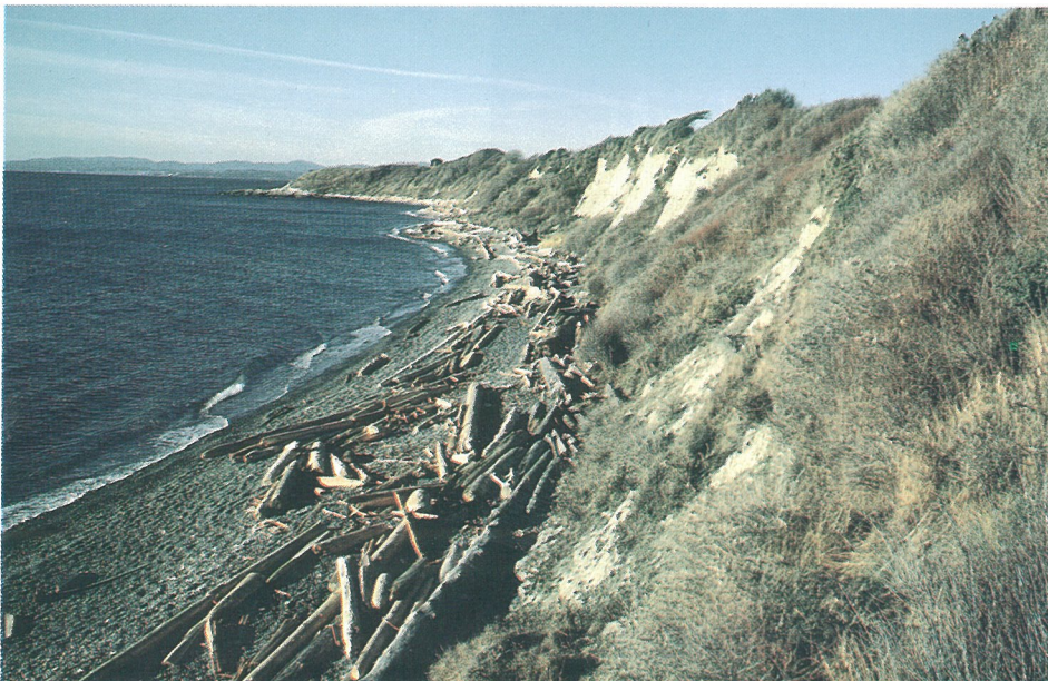
Steep, exposed soil banks are susceptible to coastal erosion
