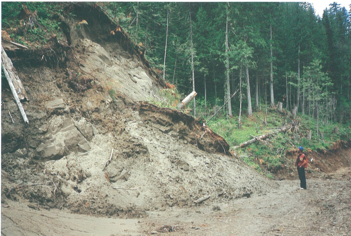
An example of a small earth slump in a glacial lake deposit whose toe was undercut by a road
