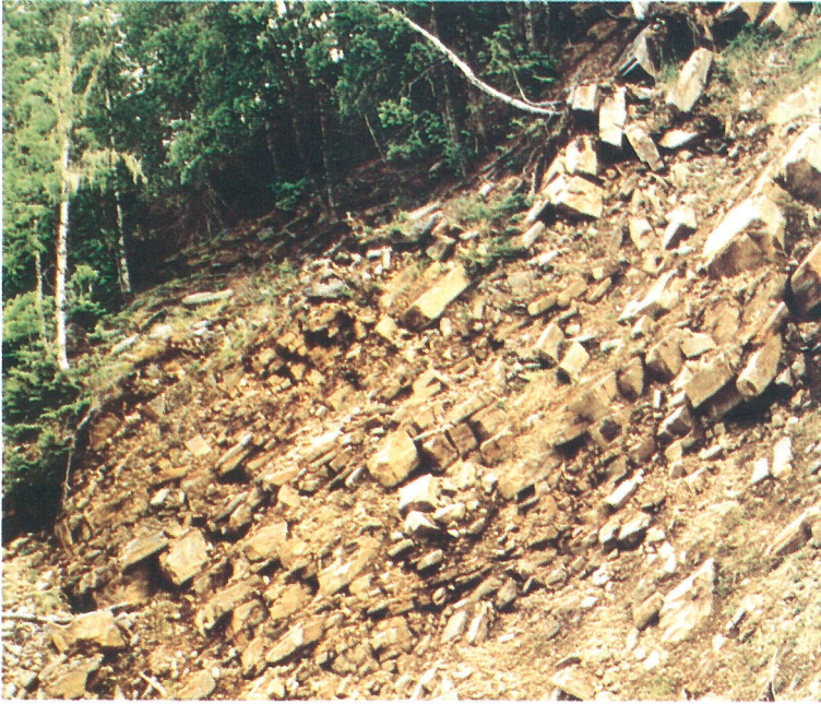
Steep fractured bedrock face
