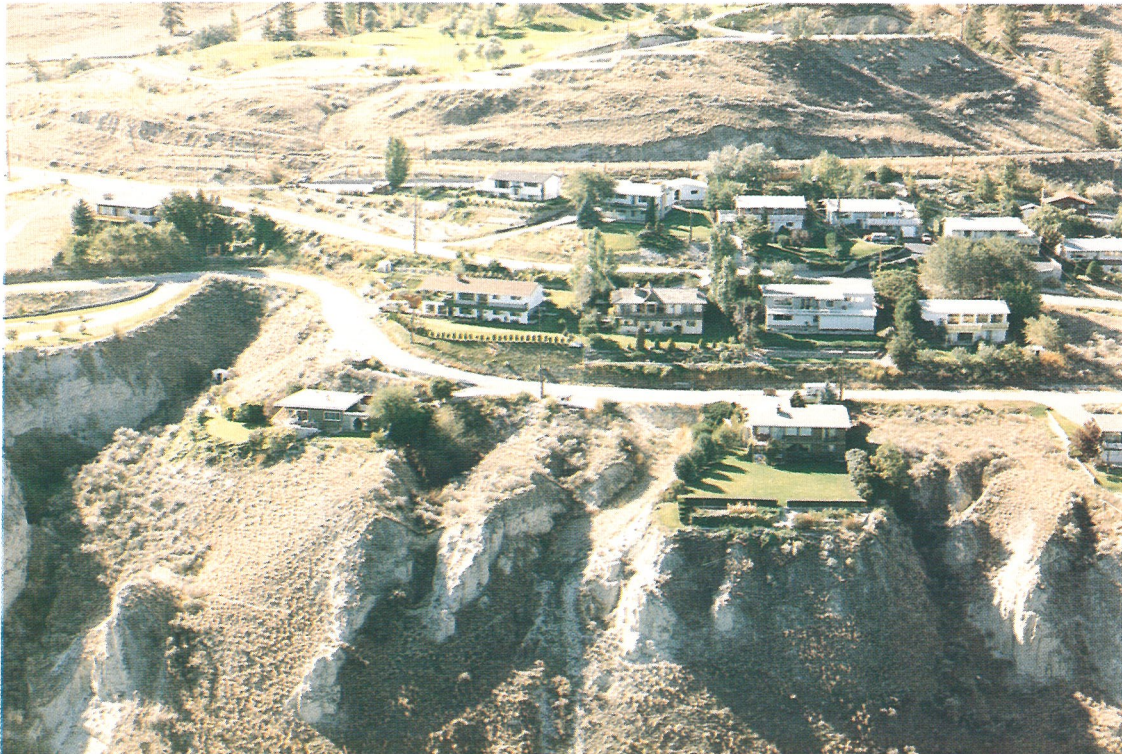
A subdivision constructed on a glacial lake silt terrace in the Okanagan
