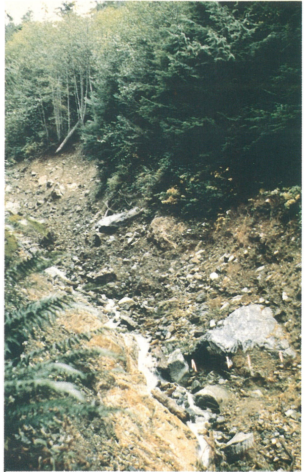
Trim lines indicate the occurrence of a debris flow
